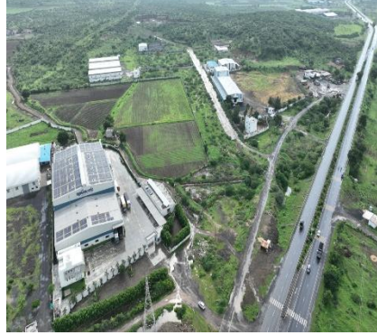
SIPL Plant Aerial View
